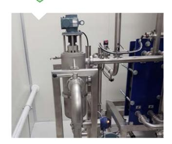
Rotary filter auto dump with automatic pressure differential pneumatic valve. Control box, o-10 bar digital pressure gauges and 10-amp single phase plug.
