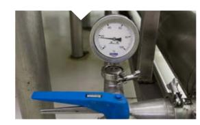
Temperature gauge with 1 ½" tri-ferrel connection.
